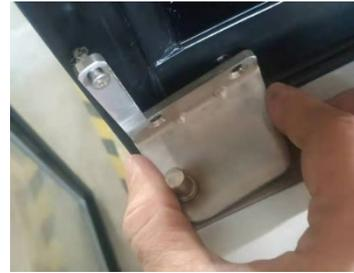
3. Turn the door 180° and put it onto the left side lower hinge and hold it at close position.
